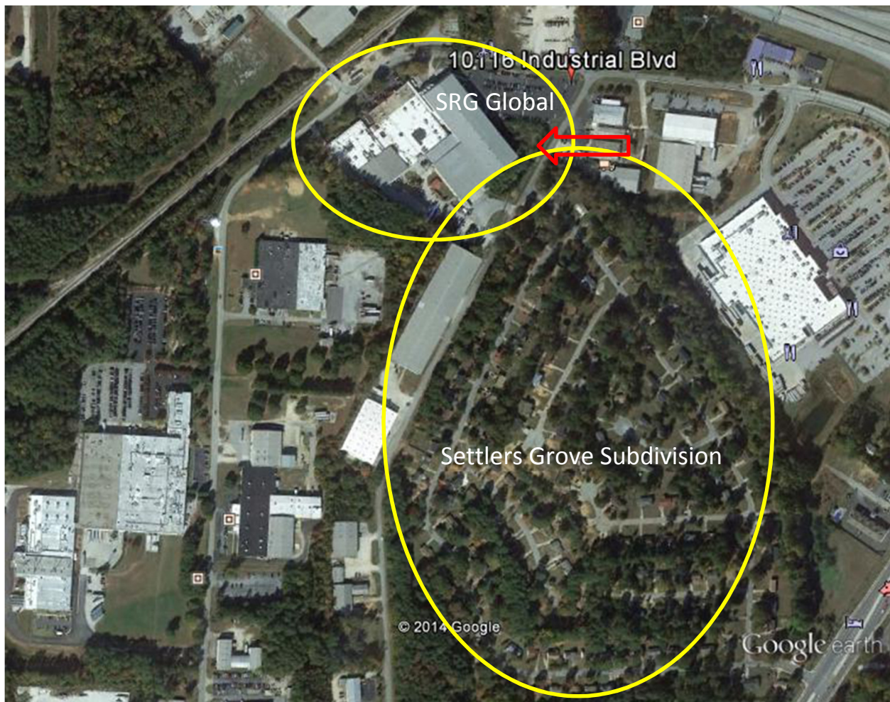
Figure 1: Aerial photo of the SRG Global manufacturing plant (top of photo) and the Settlers Grove subdivision southeast of the manufacturing plant. The red arrow points to the sedimentation pond, which can be seen on the eastern boundary of the manufacturing building adjacent to Hazelbrand Road. The sedimentation pond is overgrown with vegetation. The entrance into the Settlers Grove Subdivision on Waterford Road can also be seen directly across the southern-most section of the sedimentation pond.
