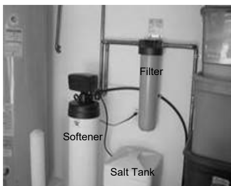
Water Softener and Filter Installation
