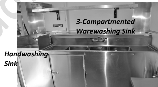
"Mobile Catering Unit Combination Warewashing 3-Compartment Sink and Handwashing Sink"
