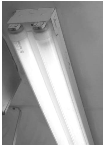
"Plastic Tube and Cap Shielding Installed"
