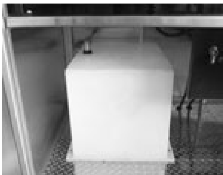
“Permanently Mounted Plastic Potable Water Storage Tank”
