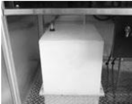
“Permanently Mounted Plastic Potable Water Storage Tank”
