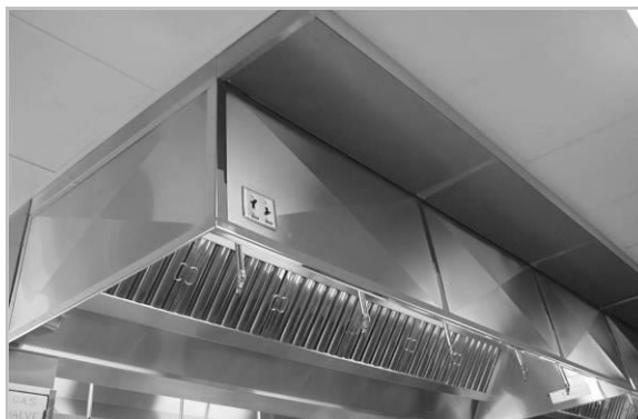
Island Hood Installed Over Cook Line
