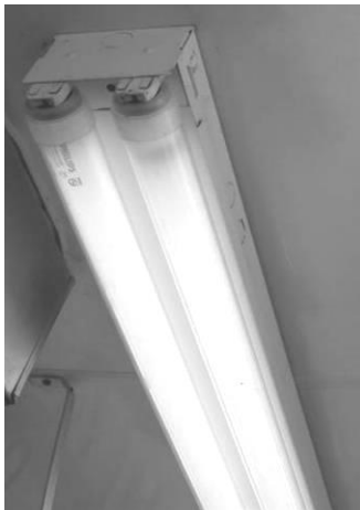
"Plastic Tube and Cap Shielding Installed"
