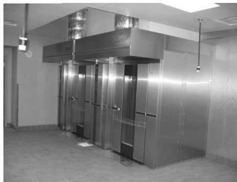
ILLUSTRATION Q-6 Eye Brow Hood on a Conveyor Oven
