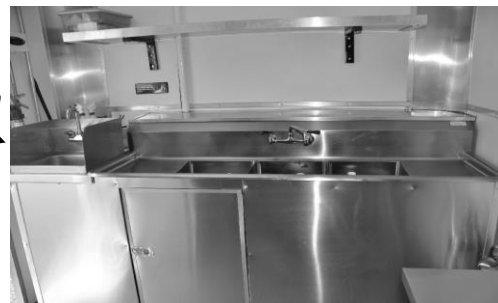
"Mobile Catering Unit Combination Warewashing 3-Compartmented Sink and Handwashing Sink" and Handwashing Station
