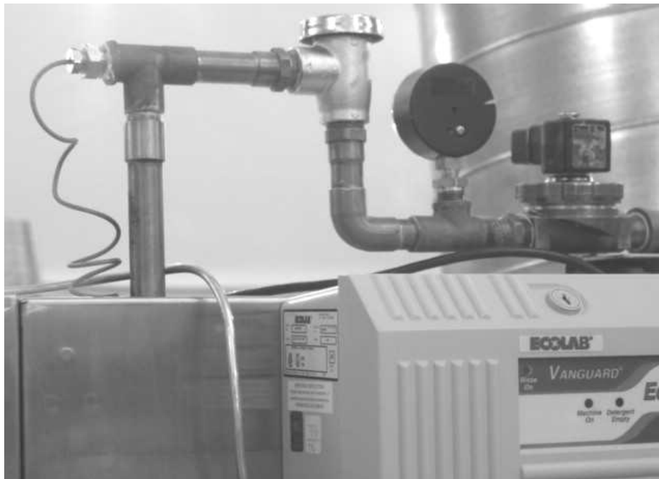
Point of installation of dispensers
