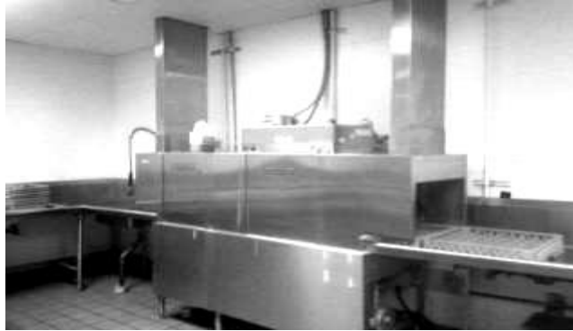
Dishwasher with Heat and Water Vapor Exhaust System
