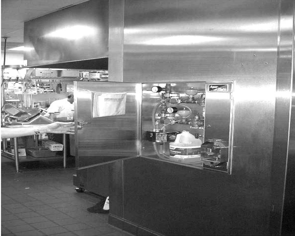
*The open cabinet of the above self-cleaning (or Waterwash Hood) ventilation hood reveals the automatic cleaning unit apparatus. Notice the cleaning agent in the visible jug that is connected to the cleaning unit. Instructions on how to operate the self-cleaning unit are located in the pouch on the cabinet door.*
