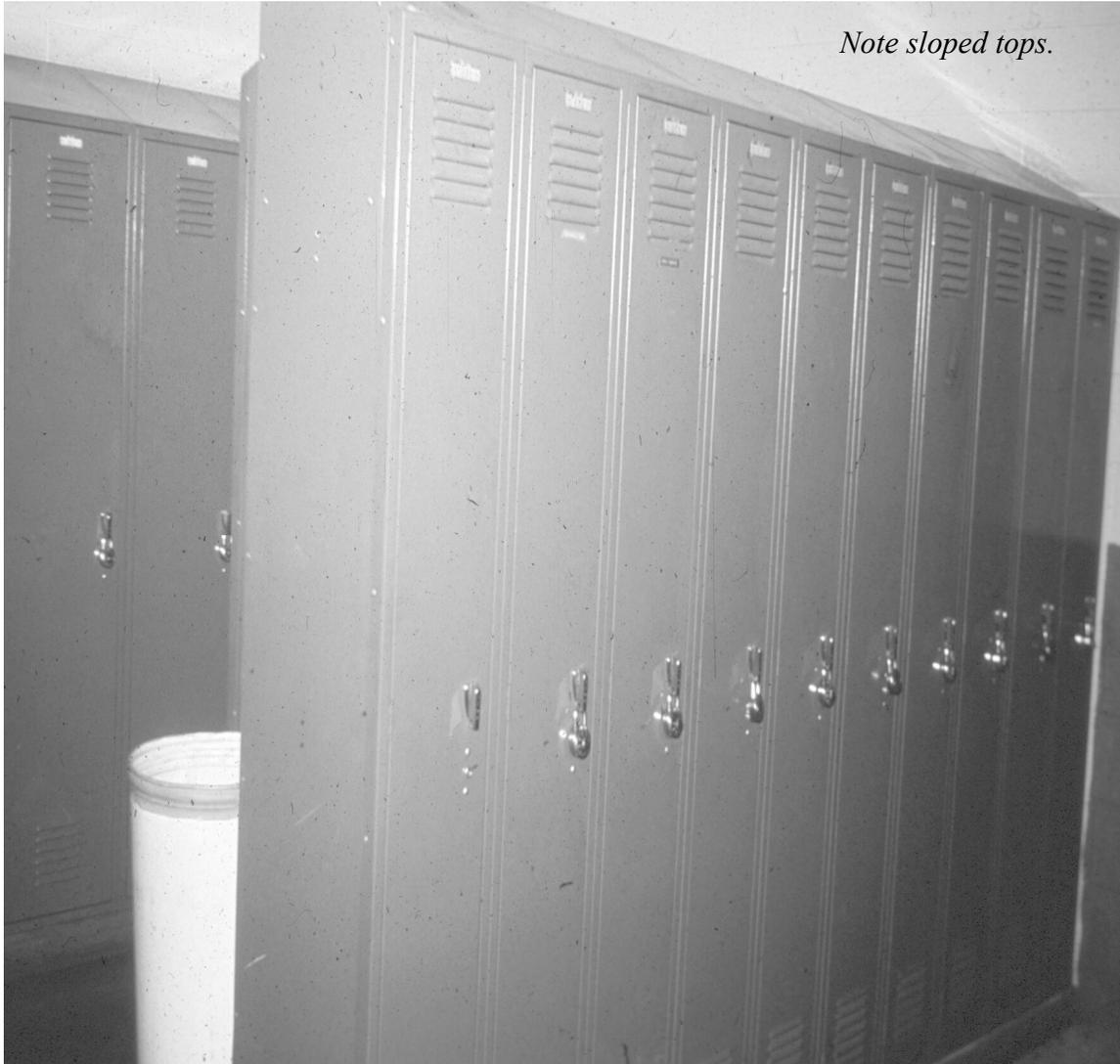
*Sloping tops of lockers provide for the determent of the collection of debris and vermin harborage.*
