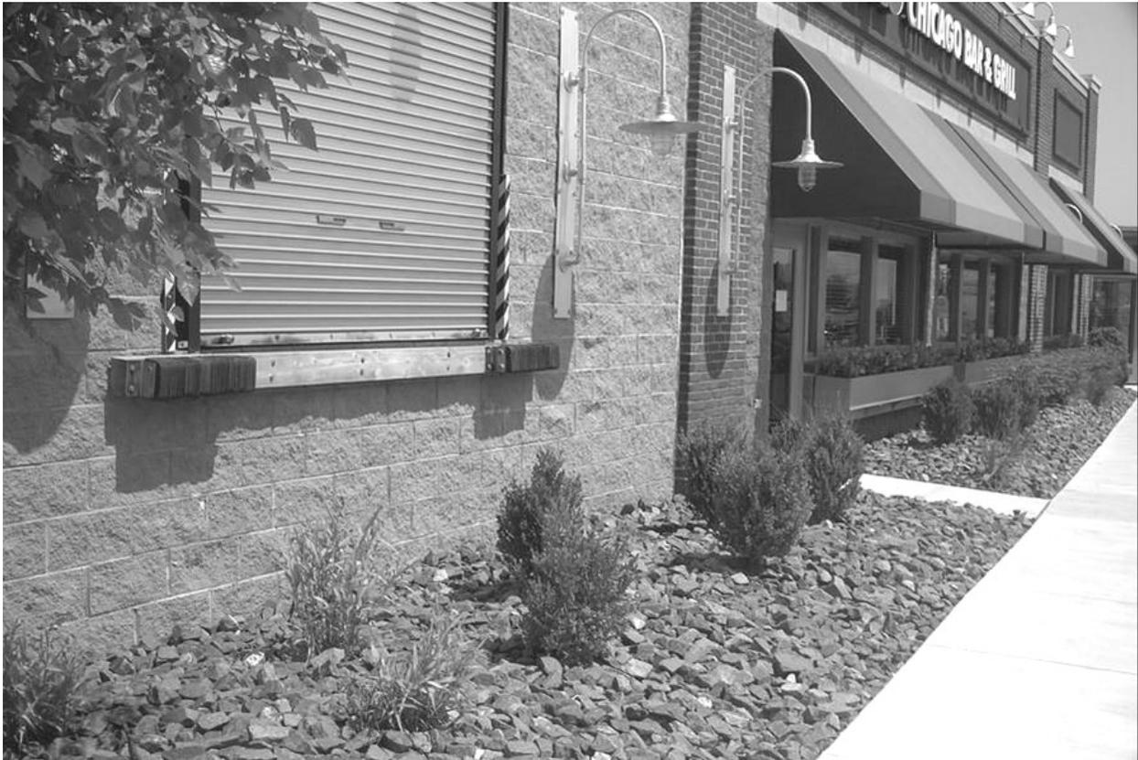
*Outside landscape material should be small enough not to create void spaces for pests to travel and hide. Shrubbery and trees should be kept at a minimum and away from the building if possible. Loading and supply areas such as the above cargo bay door need special consideration when examining the type of flashing or other gasket type finishes are installed.*
