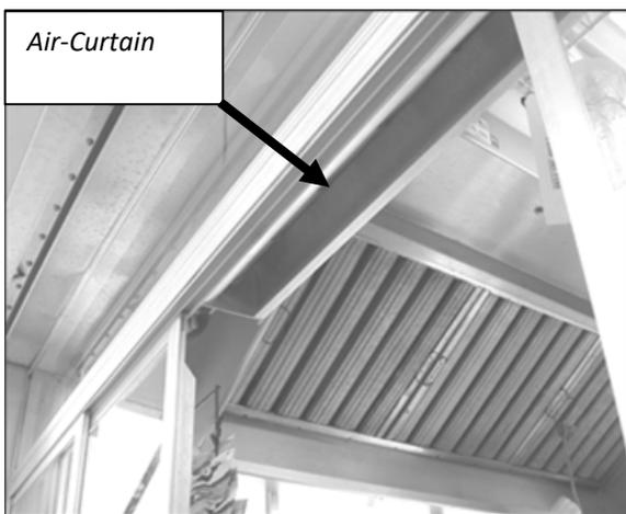
This service window has an air-curtain along the top that blows down and outward. This unit has a dropdown lid for protection during travel and periods of non-operation similar to Example "B".
