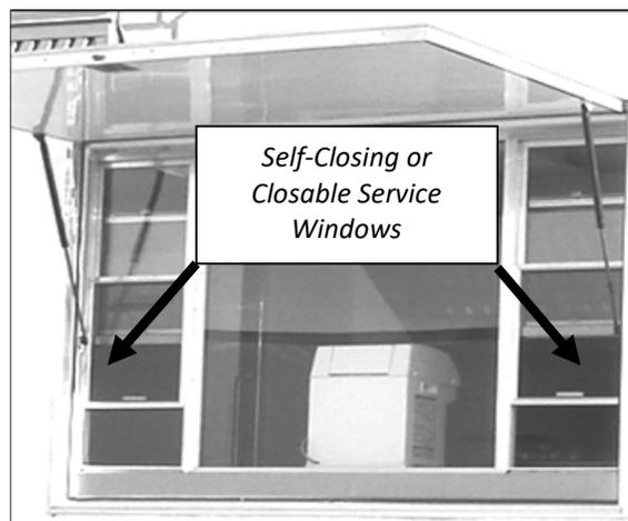
This service window design is self-closing or can be closable. Notice the dropdown lid for protection during travel and periods of non-operation.
