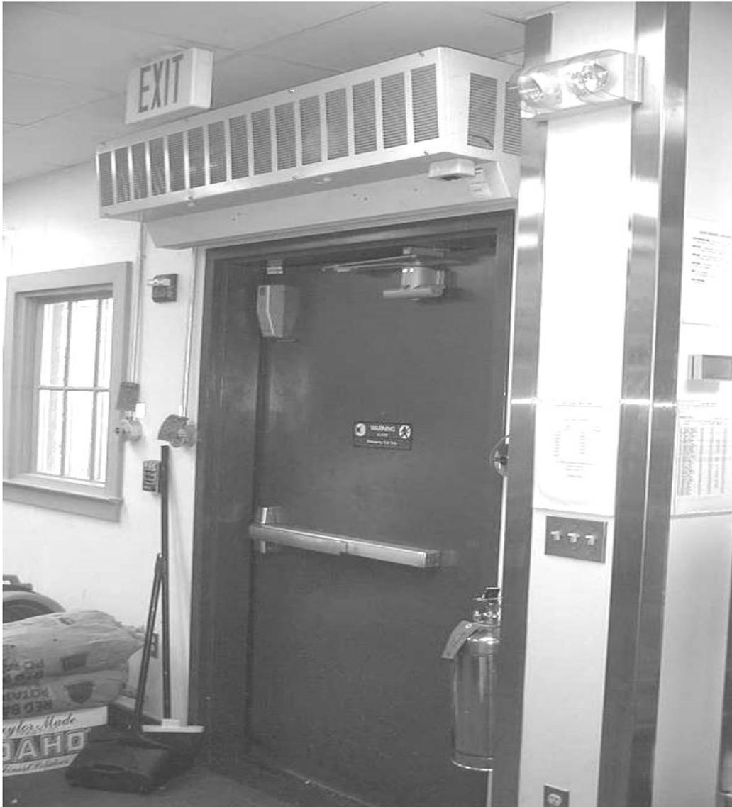
3. *Air curtains, whether installed over drive-through windows or doorways, must be sized for the opening to be protected against flying insects. These units must be auto activated whenever the door or window is opened. Air currents must blow downward and slightly outward. The units must be wired to the switch box directly so the unit cannot be deactivated at the door.*
