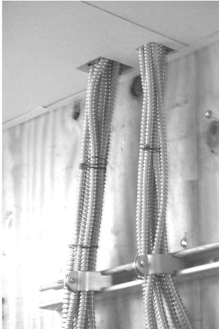
*Mechanical rooms and conduits areas are sometimes overlooked and are easy access points for most pests. Openings around conduits leading into walls or ceilings must be sealed off.*
