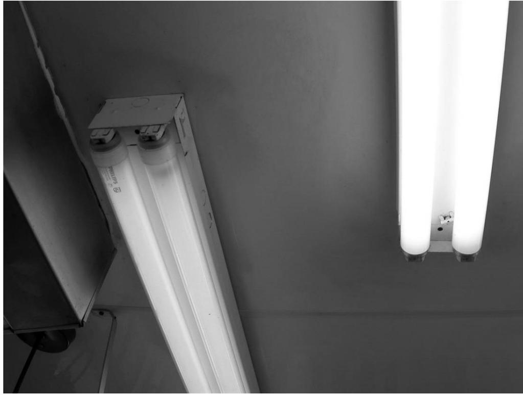
*Light bulbs must be shielded in all food service establishment except as provided for in DPH Rule 511-6-1-.07(2)(i)2. Note that the light bulbs on the left have protective sleeves over each bulb, but the bulbs on the right do not. Shields help prevent breakage caused from mop and broom handles hitting the bulbs. Shields also prevent broken glass from falling when florescent bulbs burst. In this way, food, utensils, single-service and single-*
