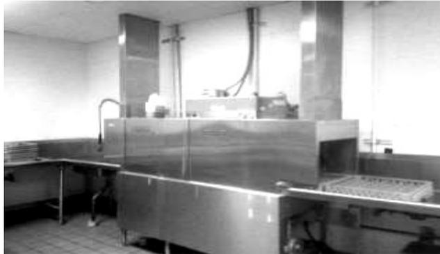
*This Type II Hood system is called a Pans Leg Hood due to the two duck work located at the entrance and exit of the warewashing machine looks like the legs of a pair of pants.*
