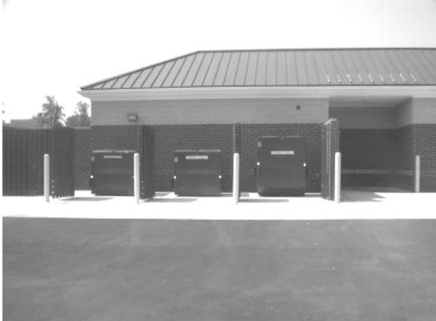
3. *Receptacles and waste handling units for refuse and recyclables such as an on-site compactor shall be installed so that accumulation of debris and insect and rodent attraction and harborage are minimized and effective cleaning is facilitated around and, if the unit is not installed flush with the base pad, under the unit. See Illustration T-5 and Illustration T-6.*
