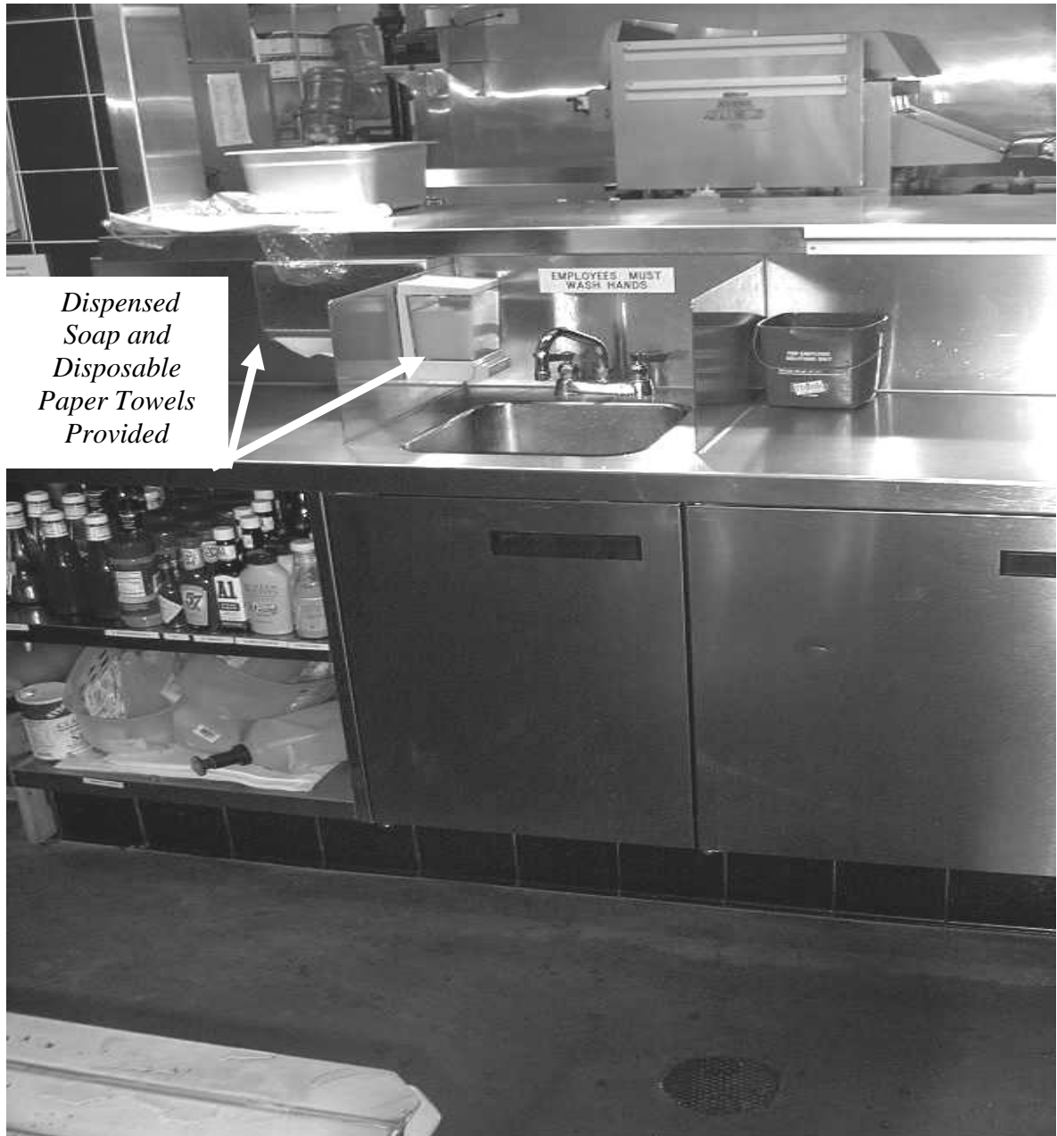
The above picture is an example of the adaptation of shielding to prevent splash from handwashing getting onto work surfaces.
