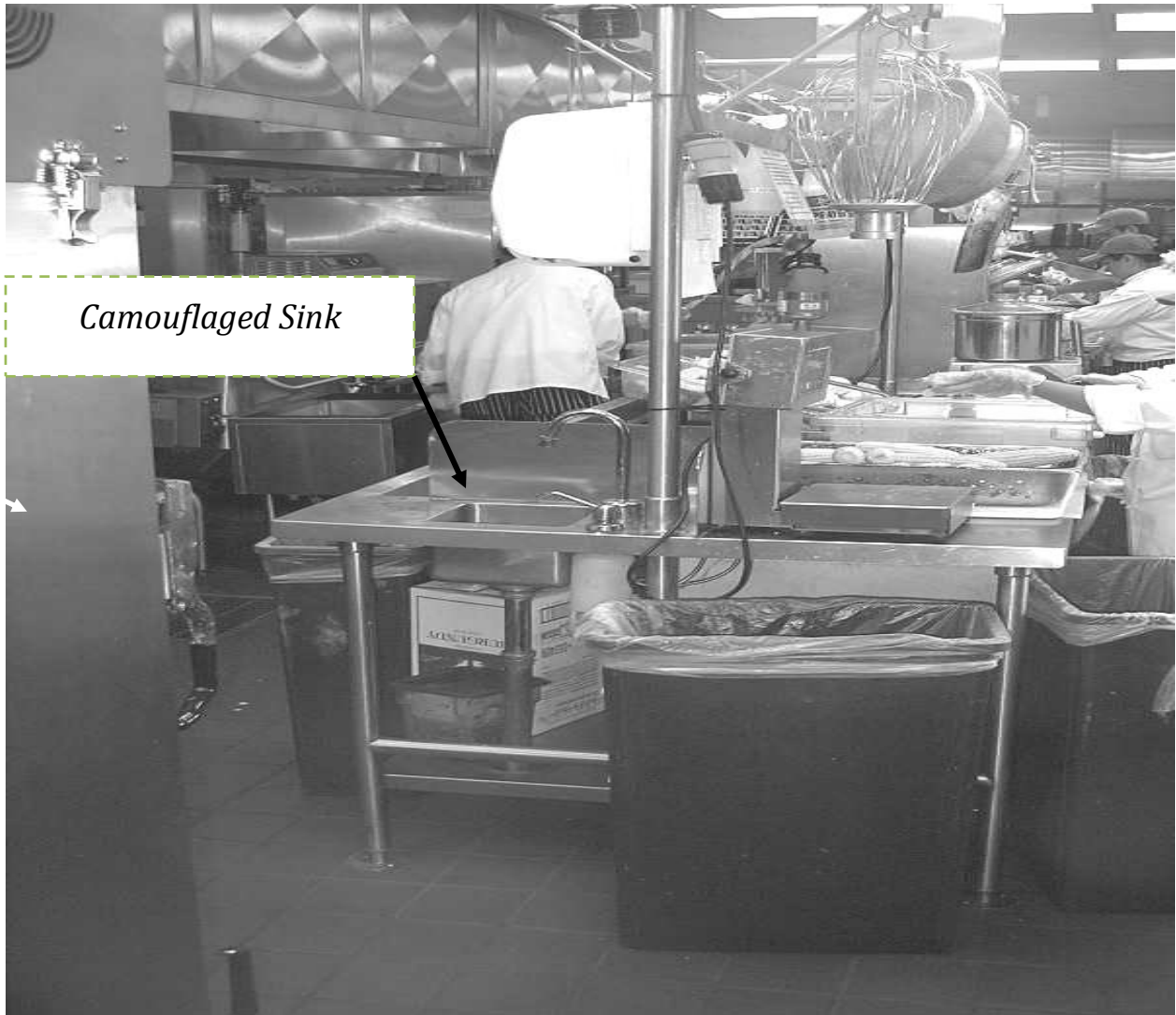
Camouflaged Handwashing Station located in the Food Preparation Area. The sink is not noticeable due to other equipment and other work stations.
