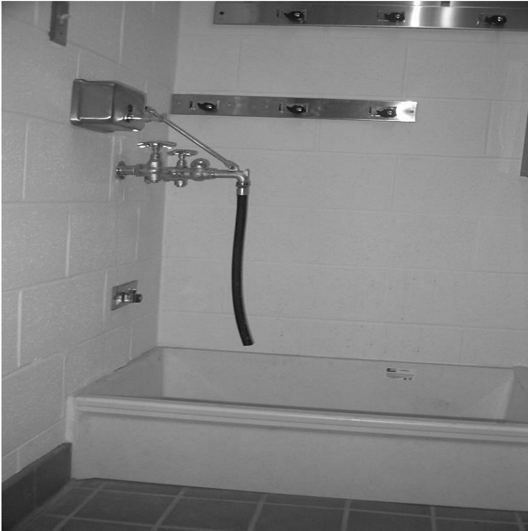
Improper use of a Utility Sink as a Handwashing Station
