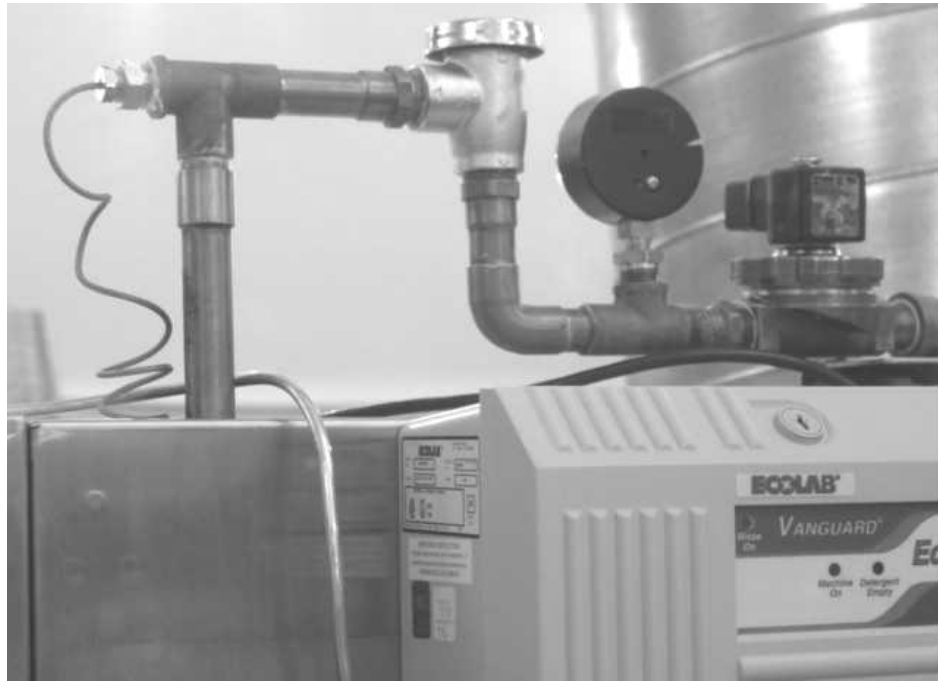
Point of installation of dispensers
