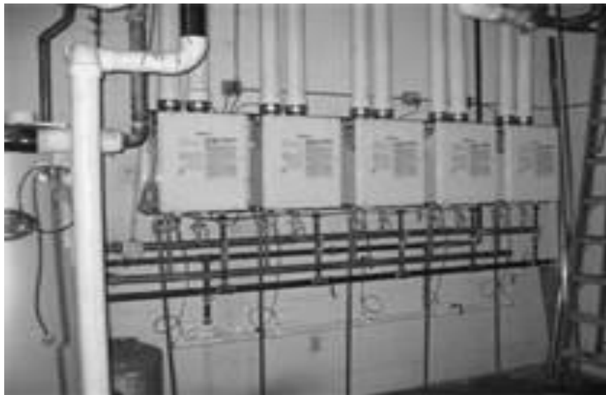
On-Demand Water Heaters in Series
