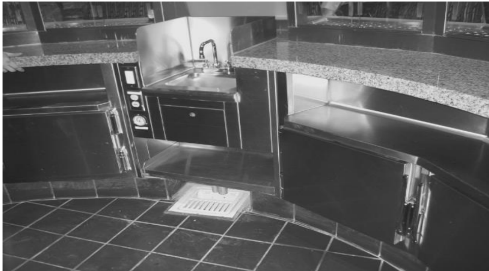
Shielded Handwashing Sink located in the Food Preparation Area.
