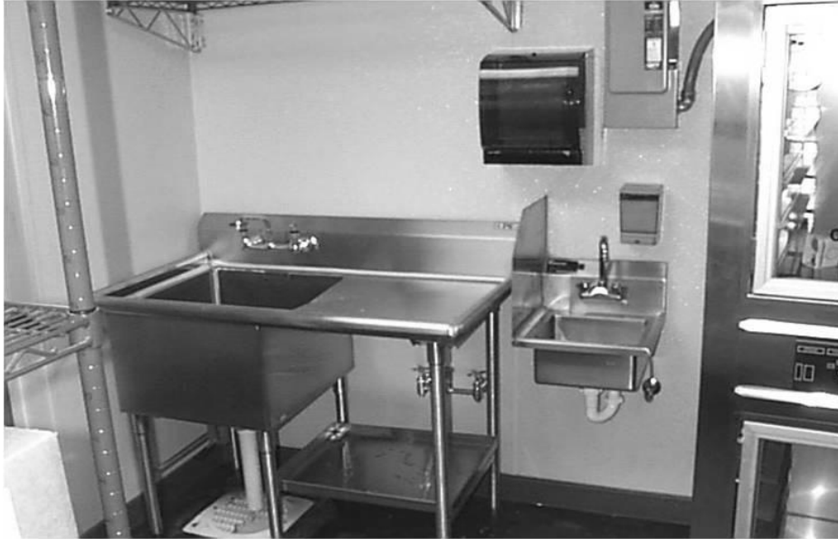
Shield Attached to Handwashing Sink providing splash protection for Food Preparation Sink
