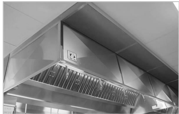
Island Hood Installed Over Cook Line
