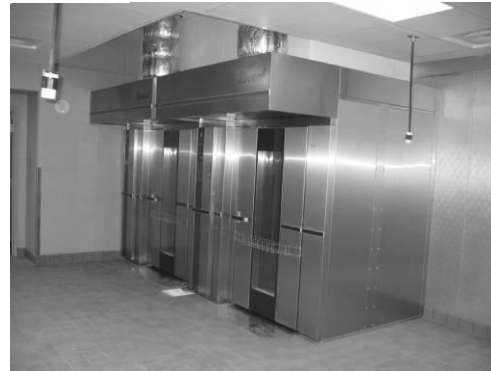
ILLUSTRATION Q-6 Eye Brow Hood on a Conveyor Oven
