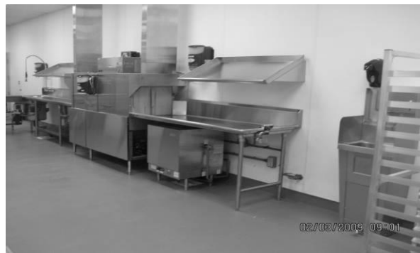
ILLUSTRATION Q-9 Typical Installation of a Canopy Hood over Warewashing Machine
